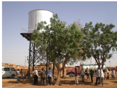
The water well and tanker
